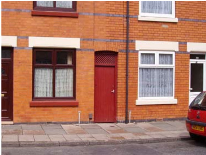
Image 3: photo showing terrace housing with gated shared access to allow bins to be kept at the rear of the property.
