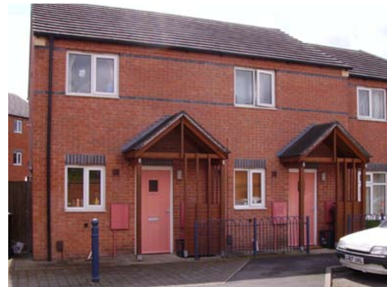
Image 5: photo showing town houses with semi-concealed bins accessible from the street for refuse collection.
