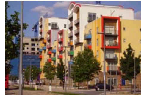
Image 15: photo showing flats providing residents with amenity space in the form of balconies.
