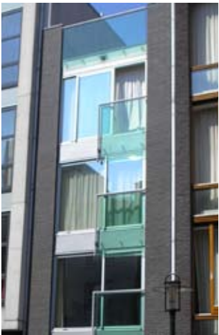
Image 13: photo shows a quality residential development with Juliet balconies. This does not substitute the need for amenity space.
