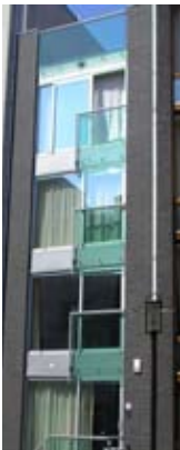
Image 29: photo shows a quality residential development with Juliet balconies. This does not substitute the need for amenity space.
