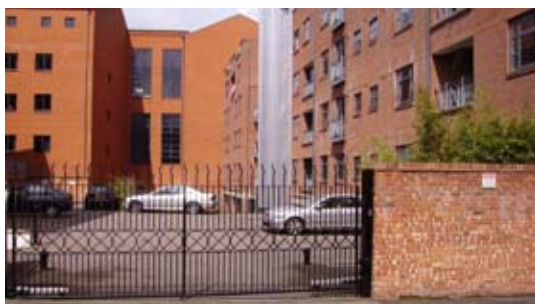
Image 16: photo showing an access gate into the rear courtyard. The space is overlooked by windows to provide natural surveillance.
