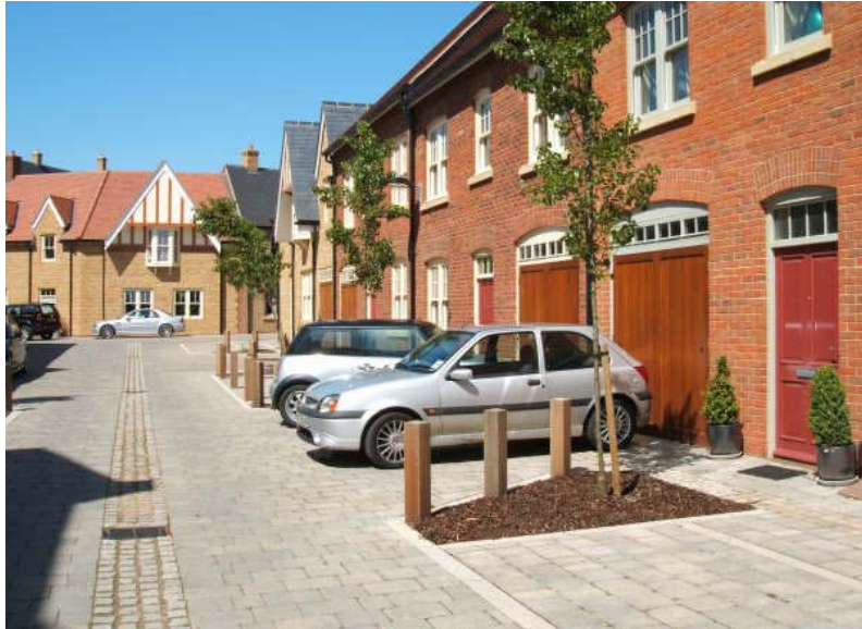
Image 41: photo showing parking arrangement at the front of the property. Photo also shows a shared surface for vehicles and pedestrians.
